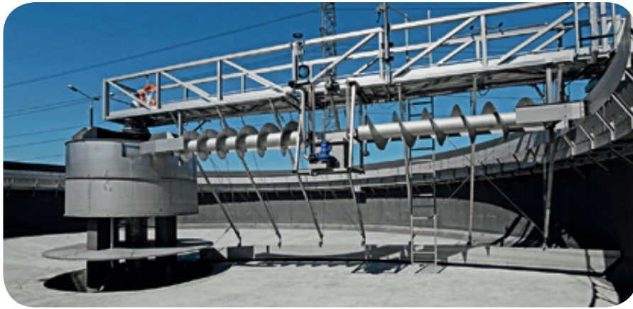
Patented screw conveyor with concentric floating extractor
