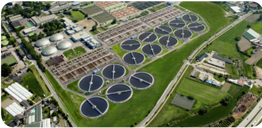
Municipal waste water treatment plant, Vienna, Austria
