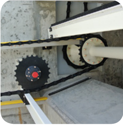
Flotation scraper made entirely of synthetic materials
