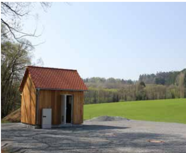
Machine house next to the plant
